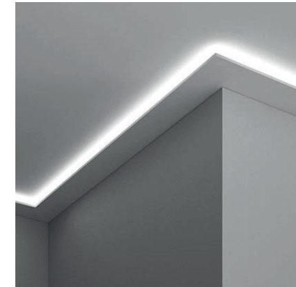
Bathroom ceiling with laminated plasterboard and perimeter LED or
